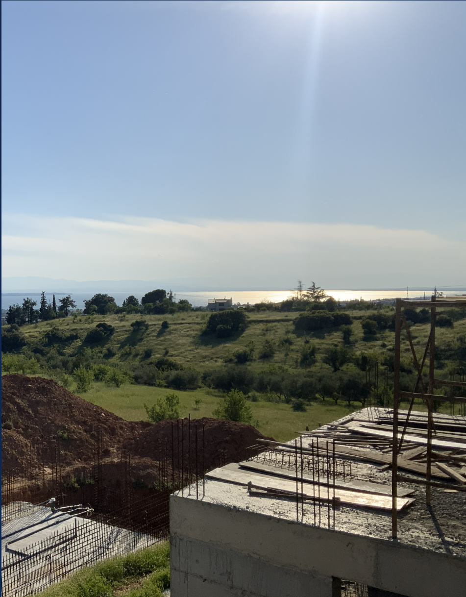
VIEW FROM THE CONSTRUCTION SITE
