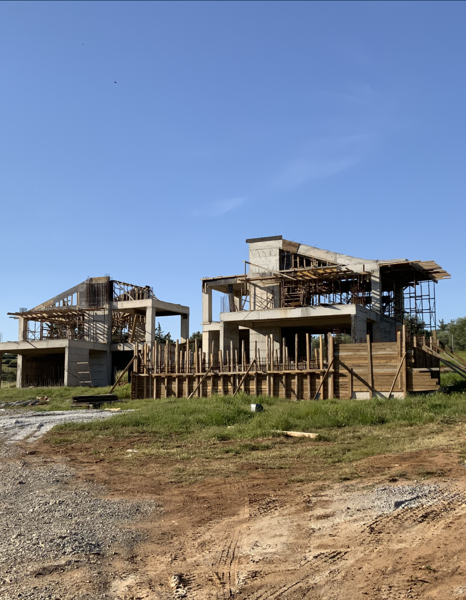
CURRENT STRUCTURAL WORKS
